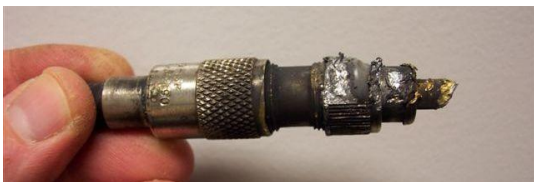
Damaged connectors? This was caused by a lightning strike.
